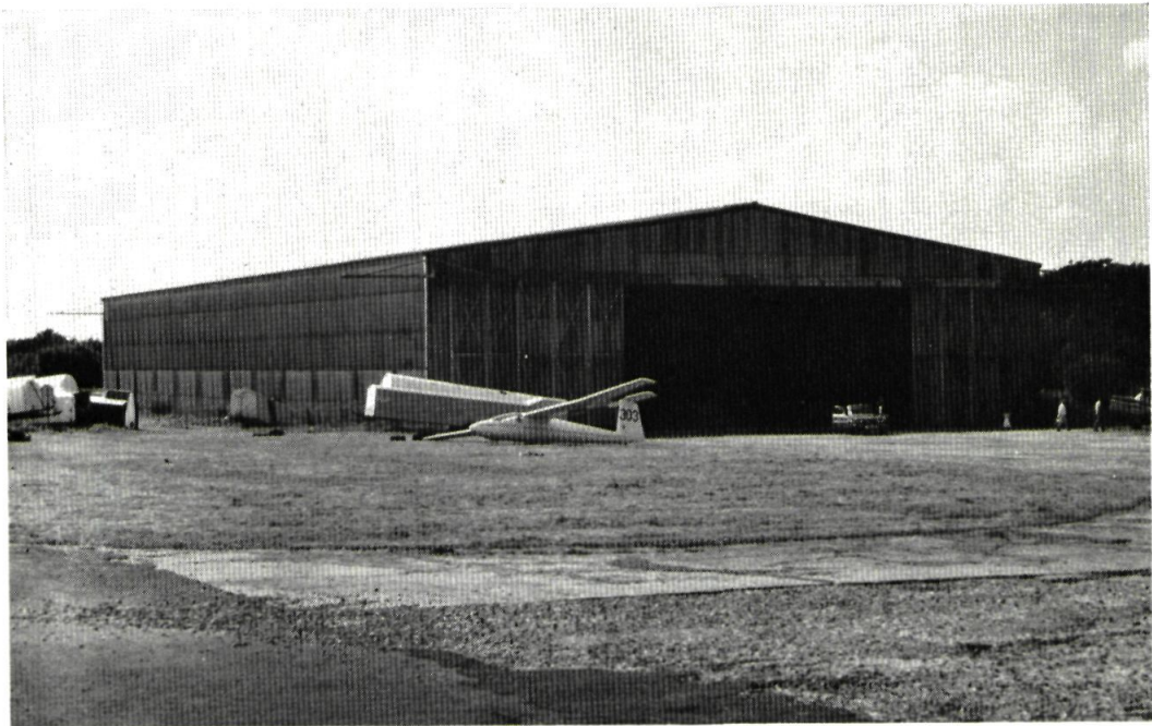
LASHAM (26): A standard T.2 hangar of 1943 vintage, now occupied by the Lasham Gliding Centre. ( Author's photograph, July 1971 )
