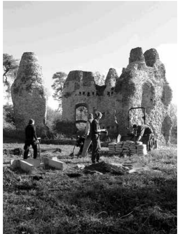
Installing the interpretation points at Odiham Castle
