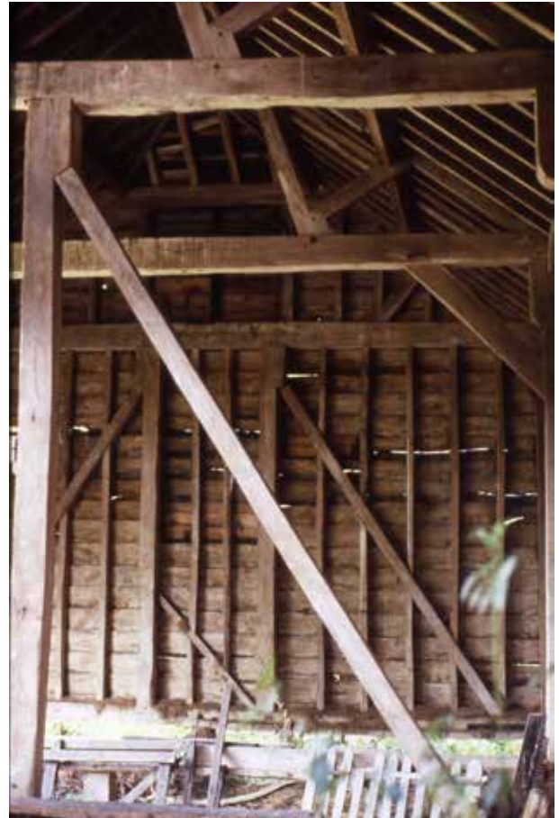
Interior photographs from 1980 showing the south-western corner of the building.
