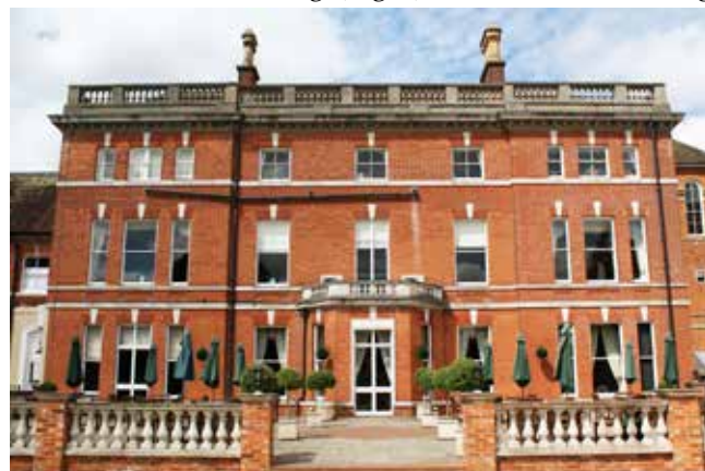
Fig 5 South-facing side of Oakley Hall showing Wither Bramston's central infilling between the two wings and Beach's third storey addition.
