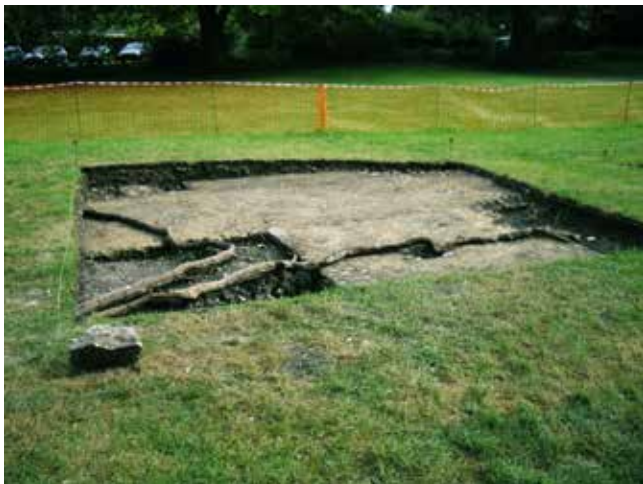
Fig 2. St Elizabeth's College, Winchester: foundations and buttresses at the north-east corner of the church
