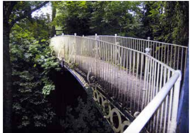
Fig. 1 The Iron Bridge, Andover
