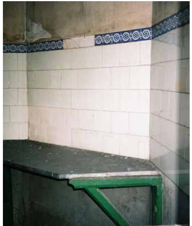
Fig. 2 Interior view showing the tiled walls and slate-work surfaces
