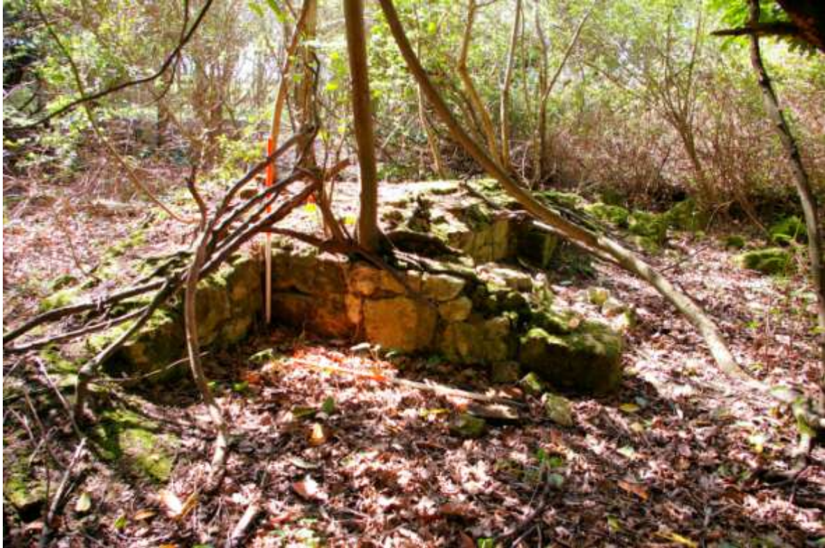
Figure 11 New House Copse: the footings of a house, constructed of large limestone blocks and brick bonded with lime mortar. The remains coincide with a dwelling first shown in AD 1868 on the first edition Ordnance Survey map. One metre scale rods (Photograph: Berkshire Archaeological Services)
