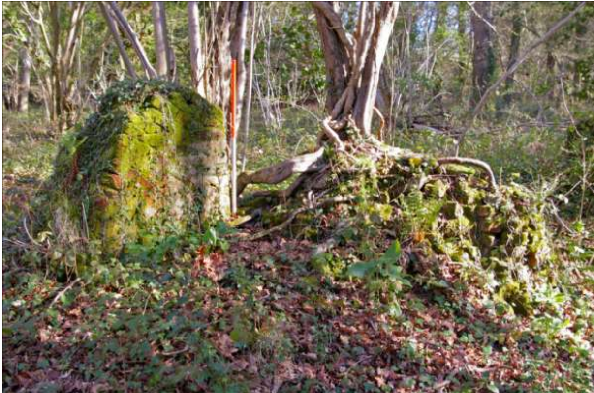
Figure 12 Whitefield Rough: remains of a brick kiln dating to the mid 19 th century (AD 1854 to AD 1868; defunct by AD 1895). The woodland floor is densely overgrown and it is possible that more of the structure survives in the surrounding area. One metre scale rod (Photograph: Berkshire Archaeological Services)
