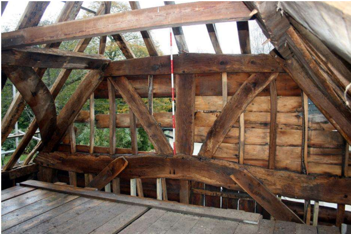
Fig. 11 'Fan truss' of the east elevation (Photograph: Souterrain Archaeology)
