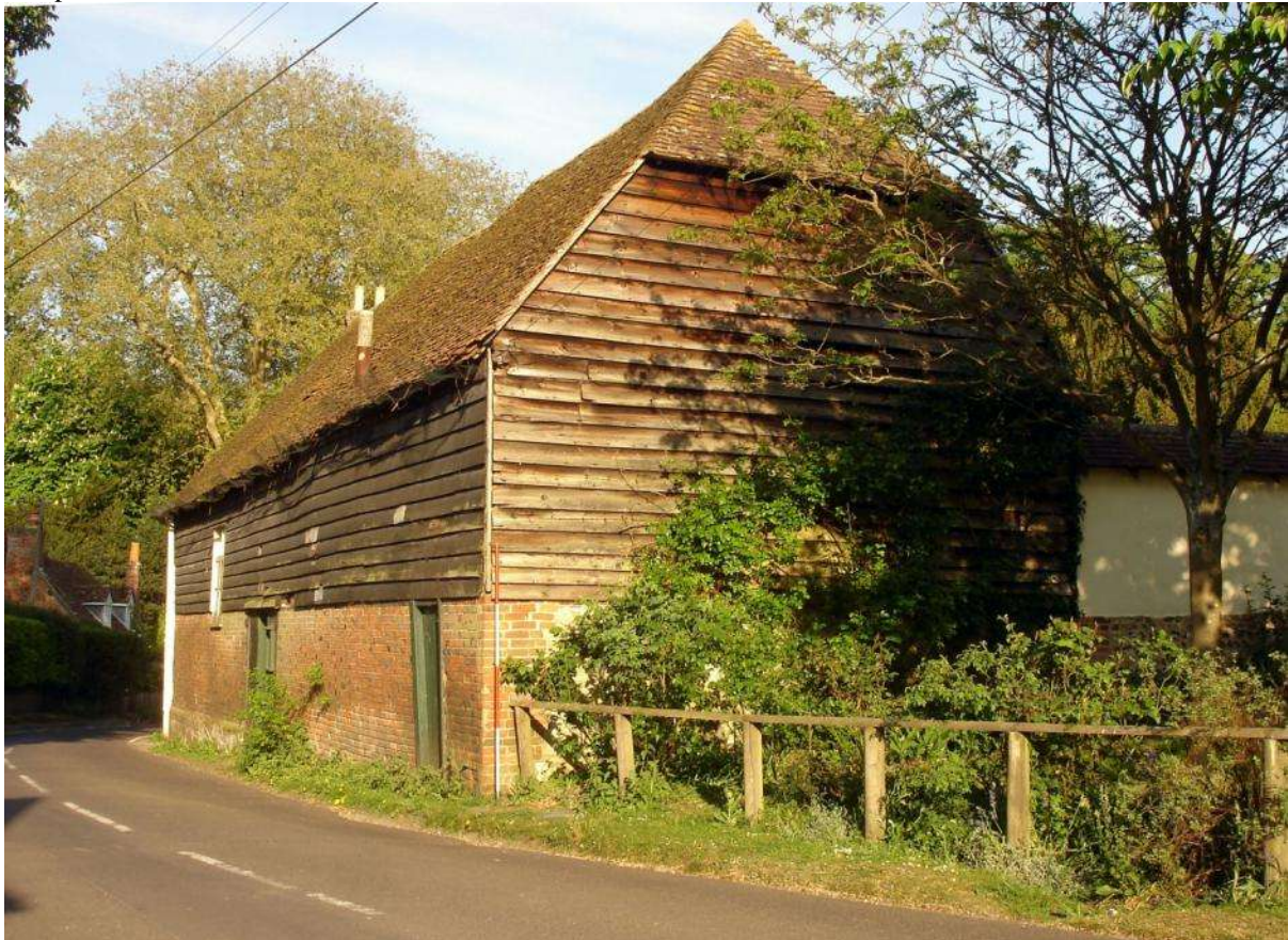
Fig 10 Mottisfont barn facing south-east (Photograph: Souterrain Archaeology)
