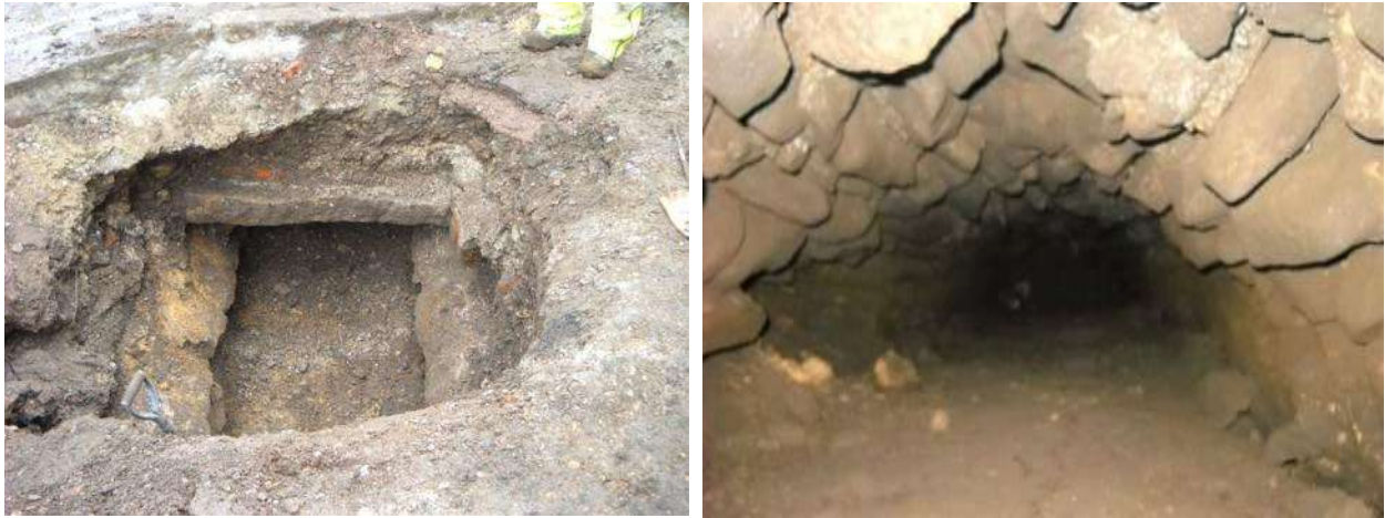
Fig 5 a&b Tunnel revealed during repaving work on the corner of Grand Parade (Photograph: Portsmouth City Council)
