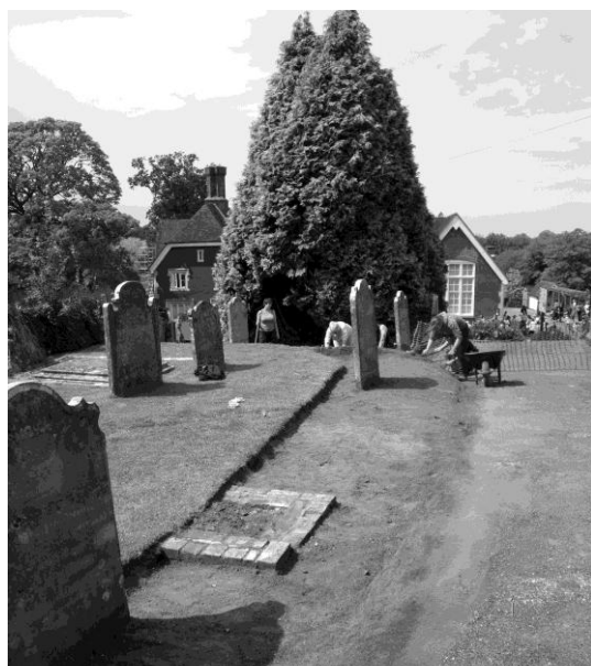
Fig. 11 Line of the new footpath and in the foreground a burial vault (Photograph: Wessex Archaeology)
