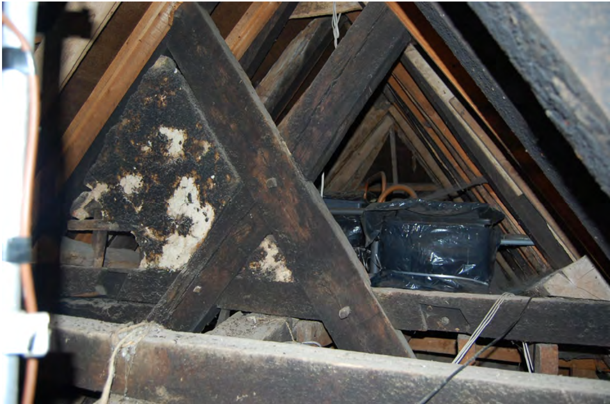
Fig. 1 Frobury Farmhouse: the roof and its passing braces
