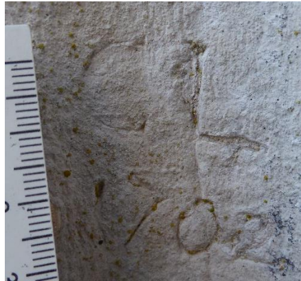
Fig 15. East side of north doorway. CL 1702
