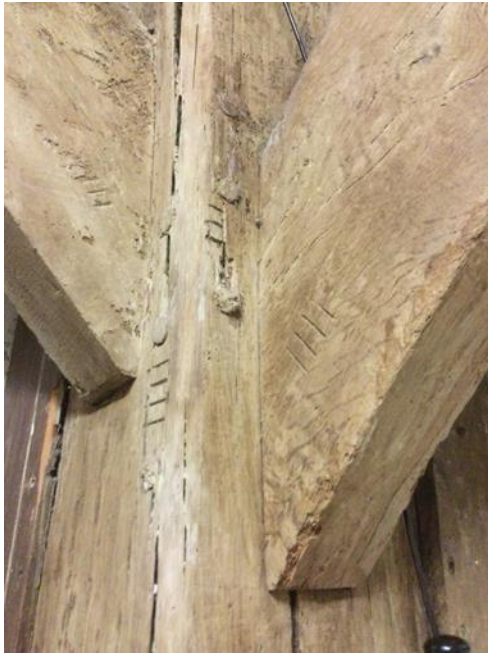
Fig 2. Carpenters' marks on post and braces in NE corner
