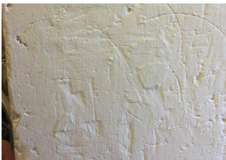
Fig 1 Ringing chamber. North window, west jamb. Intersecting circles
