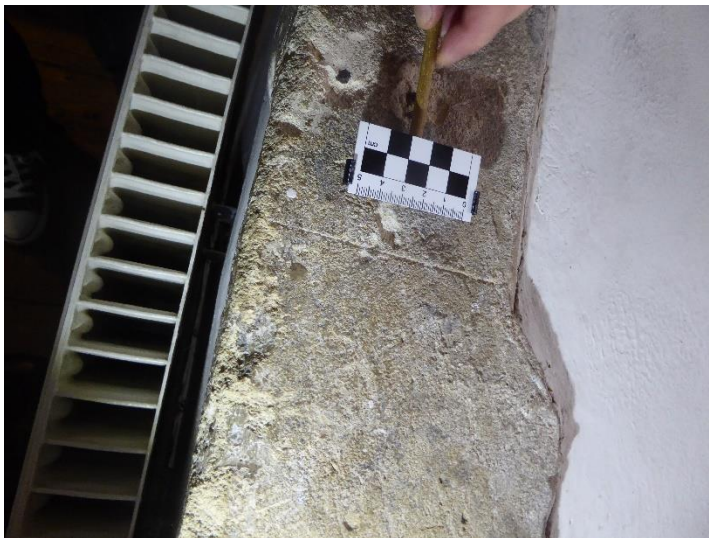
Fig 18. North window 3, sill. Mason's marking out line
