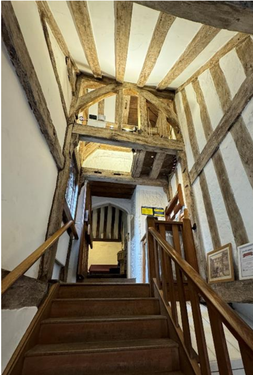
Fig 19. Timber-framed entrance staircase
