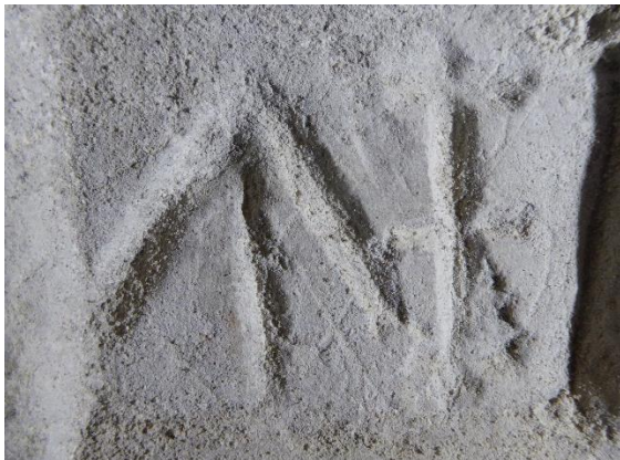
Fig 24. Undercroft, west wall. Square indentation containing graffiti arrow shape and initial I
