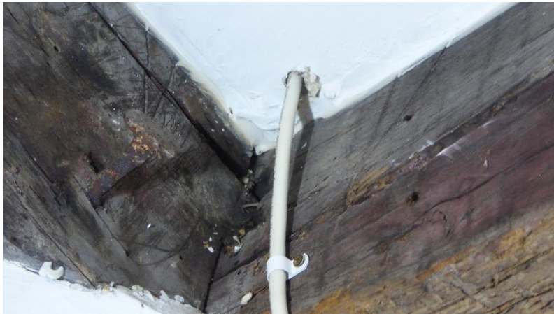
Fig 23. Carpenters' marks in vestry
