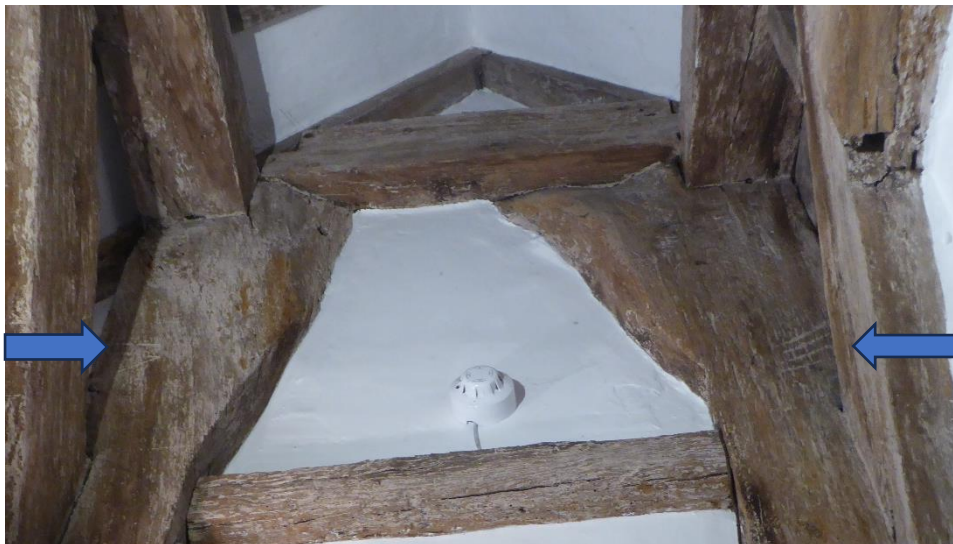
Fig 22. Carpenters' marks above north doorway. Arrows show locations on east and west sides
