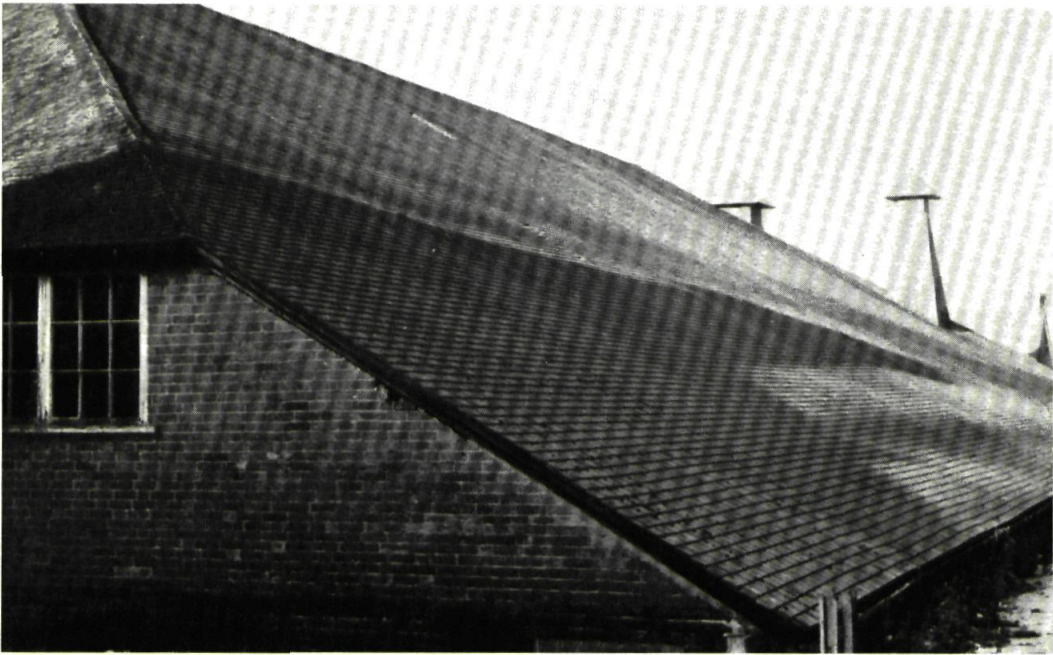
ALTON: WATNEY'S BREWERY (3); Roof of malting
