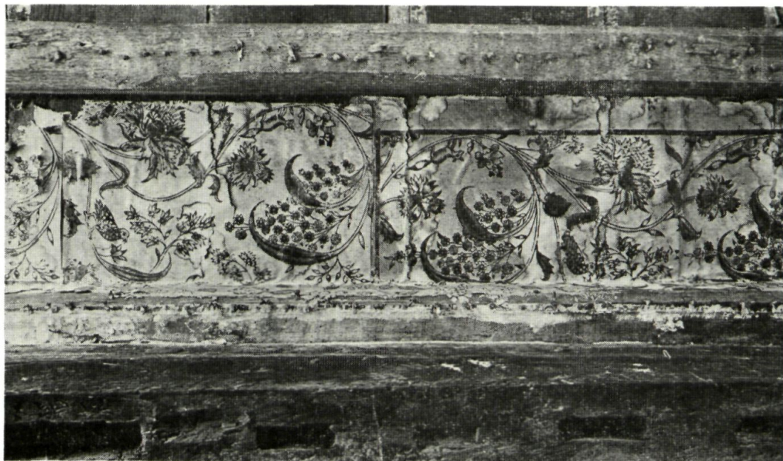
Fig. 10. Park Cottage, Swanmore. Eighteenth-century wallpaper between joists. Photograph: John Bosworth. PWCM 12482.
