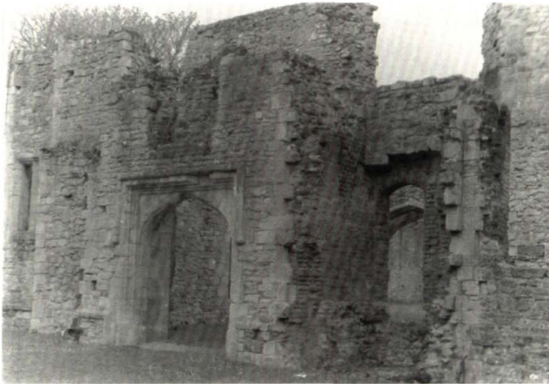
Fig 8. Entrance front of Tudor house. The doorway was flanked by two polygonal towers. That to the right shows the interior brickwork and the projecting quoins of the tower walls.
