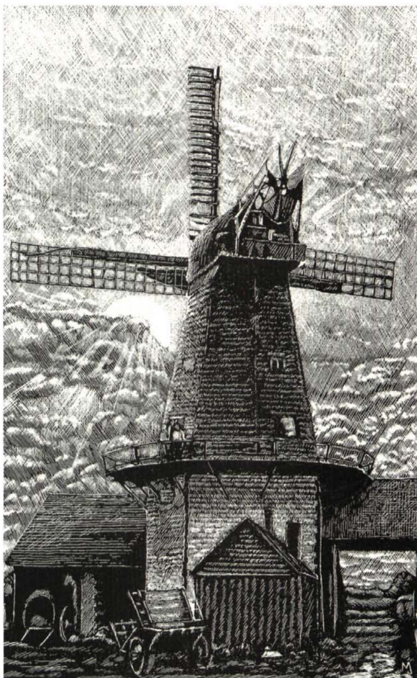
Fig 6. Weston smock mill, near Petersfield, Hampshire, was built about 1808, disused by the late nineteenth century, and the wooden tower pulled down in 1911. It had a pair of common and a pair of spring sails, which was a practical and sensible combination of sail types. (Martin Jones)
