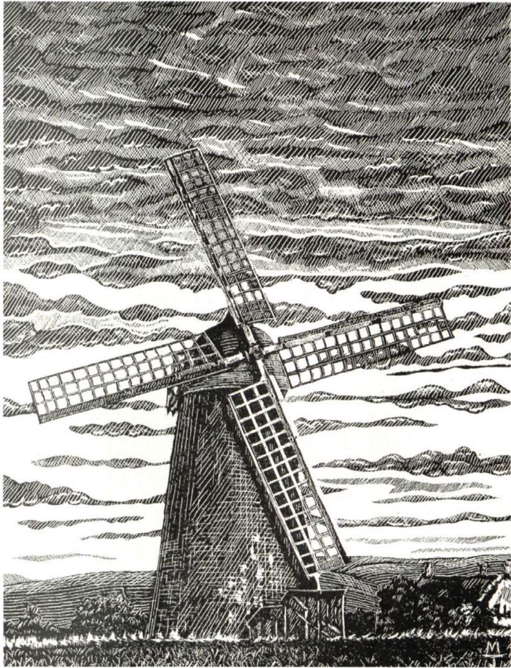
Fig 9. Owslebury tower mill, Hampshire, was built in about 1800, disused in the early years of the present century, and subsequently demolished. It had endless-chain cap turning gear and common sails. (Martin Jones)
