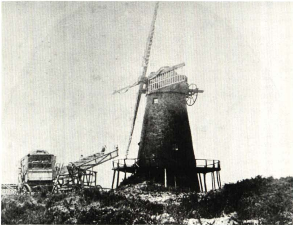
Fig 11. Bursledon tower mill in the late 1870s. The mill is clearly in regular use as the cloth sails are tied round the leading boards of the sails, and these would have been taken down if the mill was closed or not being worked for an extended period. One of George Gosling's threshing drums, and also a straw elevator, can be seen to the left of the mill. (HCCMS 0 1976.27)
