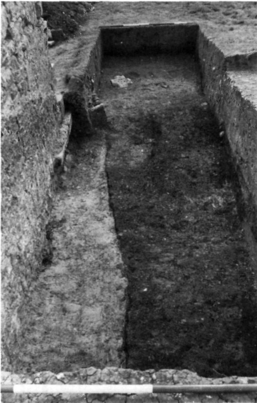
Fig 14. View west of the Aqueduct Bank under excavation. The clay-filled foundation trench is clearly visible, running at a different angle to that of the north wall of the Annexe.
