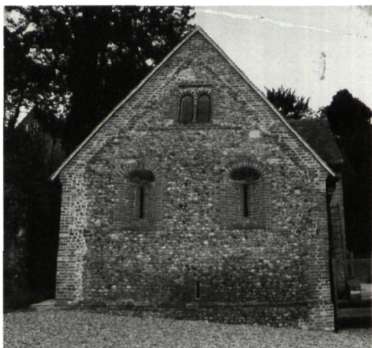
Fig 9. The north elevation of the kennels or falconry at Chawton House. The use of decorative brickwork is similar to that on the Elizabethan stables and dendrochronology suggests a similar date for this building (see text). On the three elevations still intact, there are only ventilation slits at ground-floor level but in both north and south gables are windows affording more light to a first-floor room. This room is too cramped for a gentleman's use but may have been lodgings for a kennel man or falconer.
