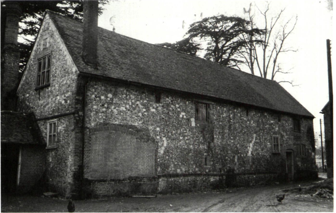
Fig 3. The north elevation of the stables at Chawton House in 1979; much more workaday than the south elevation (Fig. 2) because it faces the farmyard. The large glazed windows, the door and blocked wagon entrance were probably inserted in the nineteenth century. The ventilation slits on both floors and (perhaps) the first-floor loading doors are original (HRO 7M91/681/16).
