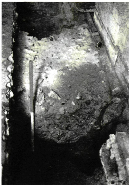
Fig. 6 Crondall Church: mortared flint wall footing from the south
