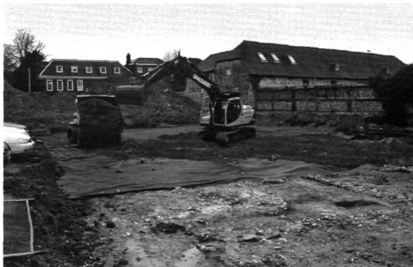
Fig. 4 Installation of the protective layer in the north-eastern excavation area, looking west
