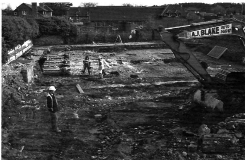
Fig. 3 The north-eastern excavation area during machining, looking east
