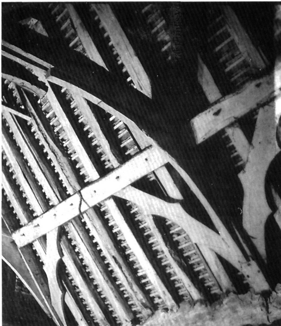
Fig. 8 Part of the roof of 1476/7 in the east block photographed in c. 1940. The cusped wind braces have not been found elsewhere in Hampshire. (Winchester Museums Service, PWCM 21500).
