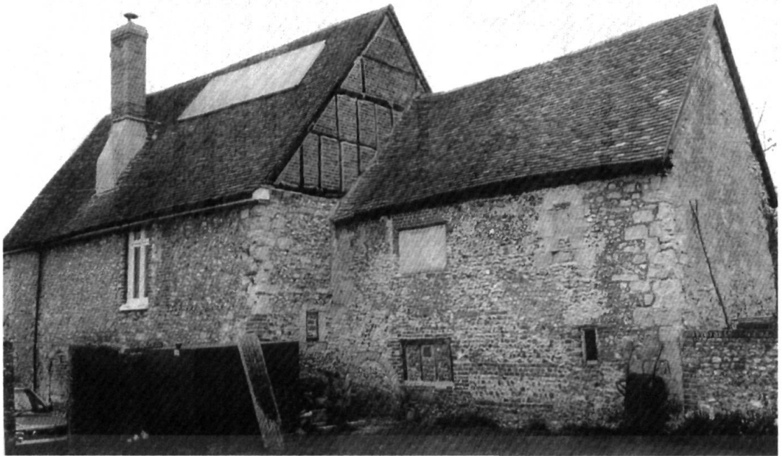
Fig. 7 The south-east elevation in 1993: just visible (bottom centre) is the round-headed arch at the west corner of the east block. This was destroyed when part of the wall collapsed in 1998 but has since been reconstructed. Note the post-medieval framing in the rebuilt gable of the larger block. (Photo: the author).
