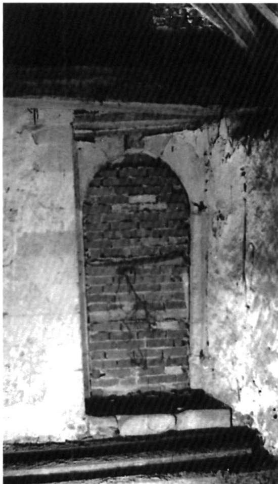
Fig. 5 The first-floor room of the east block – formerly the steward's outer chamber – photographed c. 1940. The blocked doorway formerly led from the larger, west block. Note the pintles indicating that the door swung into this room, which was in this sense an outer chamber to the larger chamber in the west block. Note also the large transverse floor joists, one of which was dated to 1244–1249. (Winchester Museums Service, PWCM 21498).
