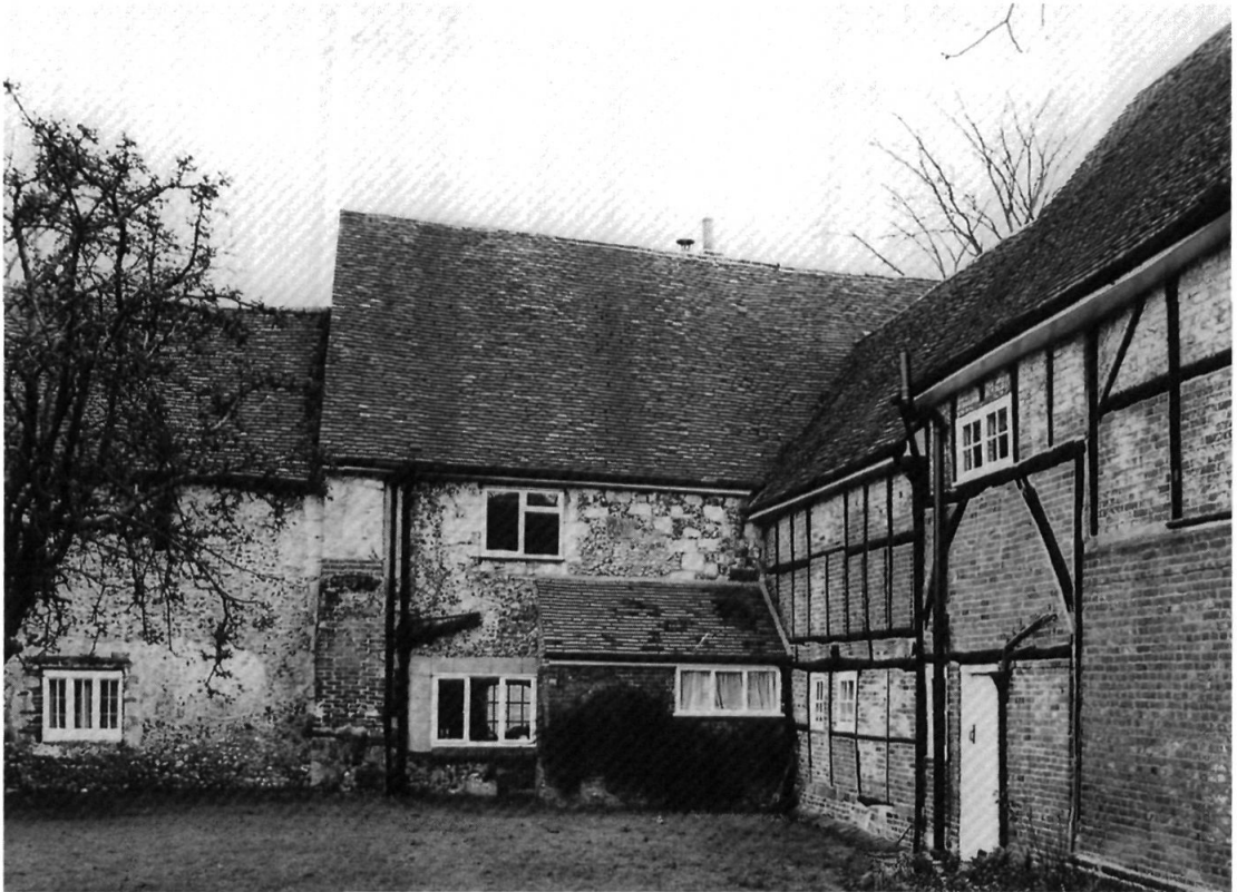
Fig. 9 Part of the north elevation of the stone-built range is on the left of this picture taken in 1984. A modern single-storey extension and adjacent window obscure the evidence for an original doorway and narrow rectangular window (see Figs 2 and 4). The timber-framed wing on the right comprises a 14th- or 15th-century bay sandwiched between two sections dating to c. 1600. This earlier bay may originally have served as a detached service room or kitchen. (Winchester Museums Service, PWCM 21510: © John Crook).
