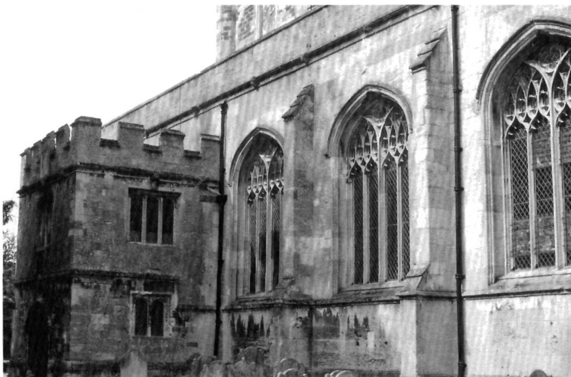
Fig. 6 South porch (c.1539) and the south aisle of nave (photo: the author)
