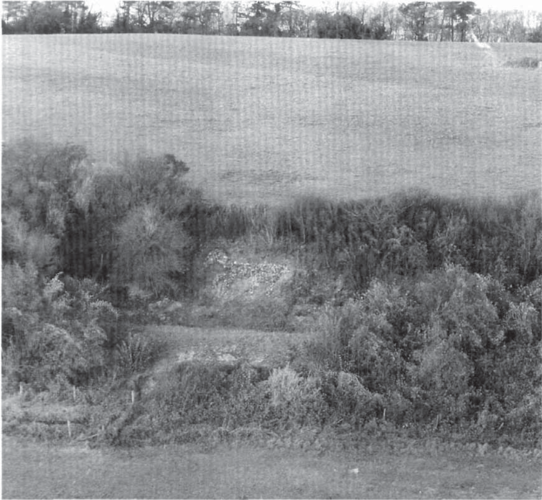
Fig. 3 The restoration completed on 23 October 2000 (author)
