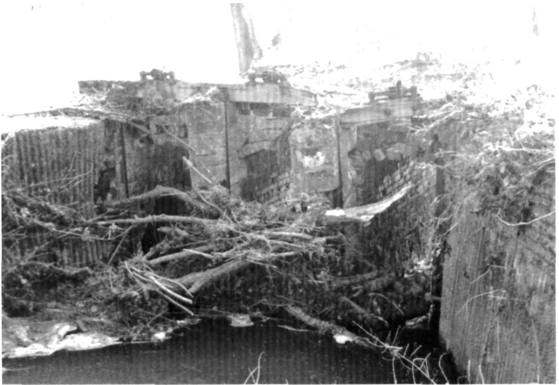
Fig. 6 The derelict main sluice on the River Blackwater
