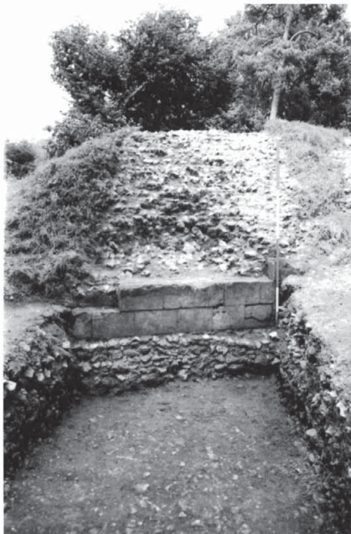
Fig. 5 The keep's mortared flint foundations
