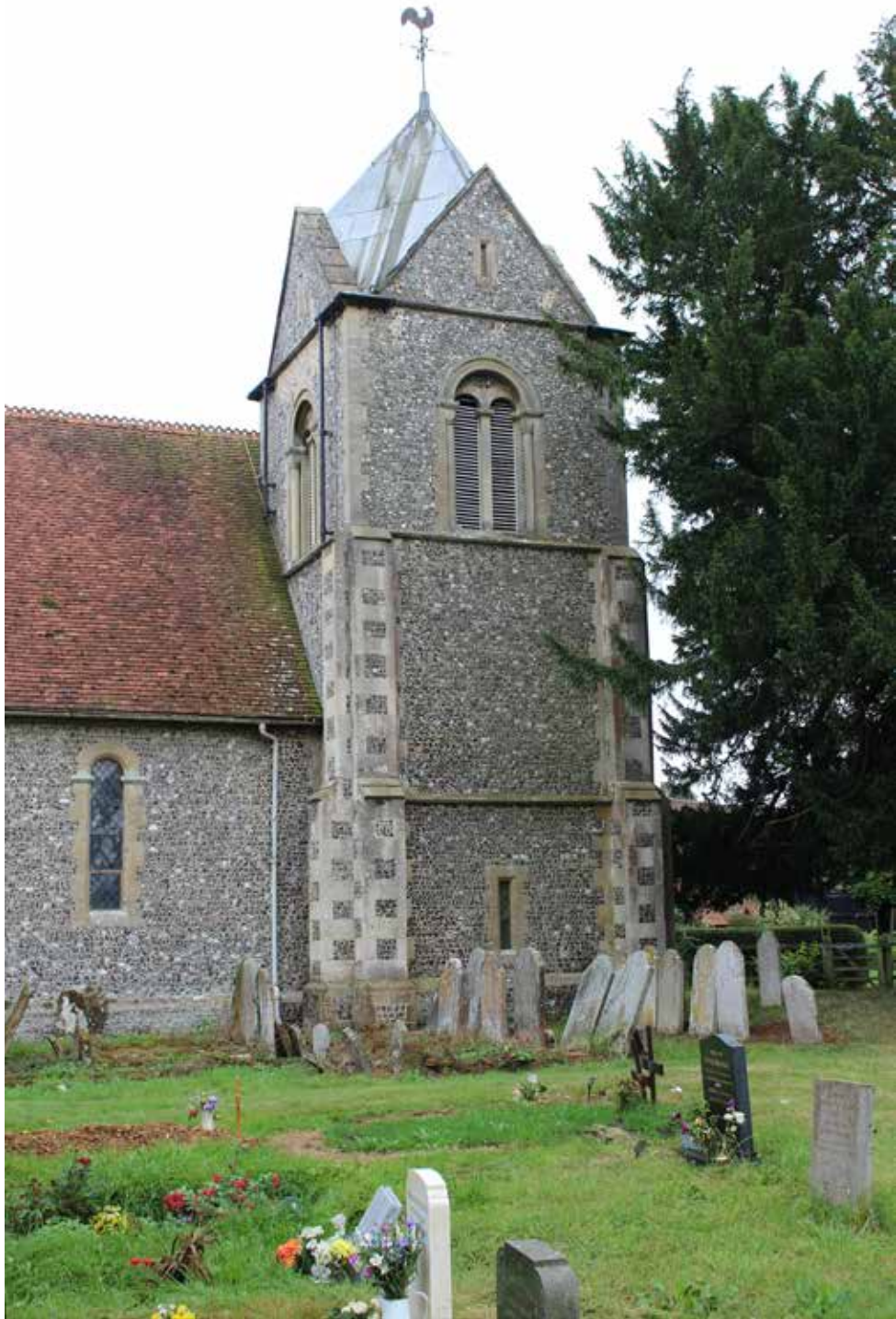
Fig. 16 St. Nicholas', Newnham from the north 2019
