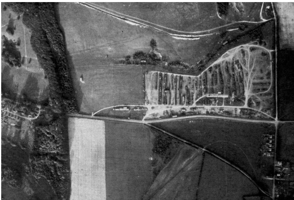
Fig. 18 Compared with the previous image (Fig. 17), this 1954 vertical relays the substantial nature of the equipment park, with the entire southern half of the area utilised. (RAF/540/1386 fr. 32 Historic England Archive (RAF Collection))
