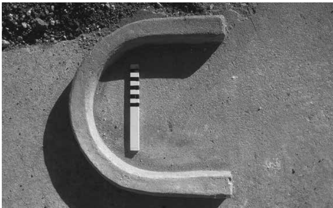
Fig. 10 An internal feature from the toilet block. This is a bucket stop and aids the correct positioning of the receptacle
