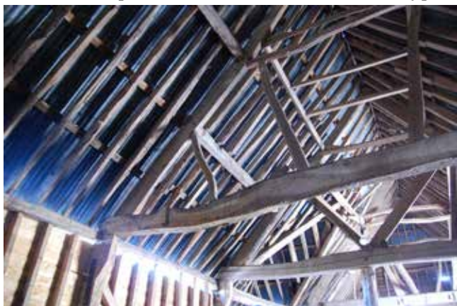
Fig. 3. The barn interior: roof trusses. (photo: Bill Fergie)
