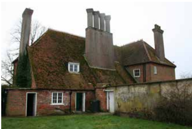
Fig. 1. Part of Upper Wyke Manor House with its Elizabethan chimney stack.
