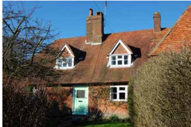
Fig. 1 No 1 Somerset's Cottages from the south. The 17 th century replacement for the original eastern bay (now within No 2) is visible to the right.
