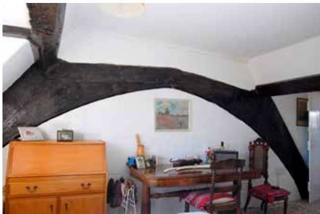
Fig. 3 Central hall truss, which would have been the centrepiece of the two bay open hall.
