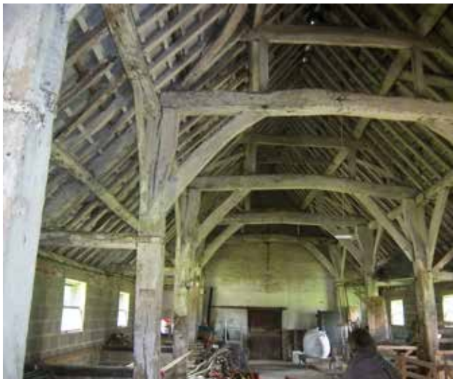
Figure 2 – Interior of Court Farm Barn
