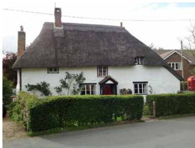
Fig 5 Abbots Rest, Chilbolton. The house was probably built in the late-16th century with a central hall heated by a smoke bay or timber chimney (seen on the left-hand side of the house in this picture). In the early-17th century a brick chimney was inserted within the smoke bay and the 'spiritual midden' was found in this chimney.
