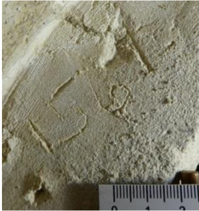
Fig 17. Clock chamber door arch. 1567
