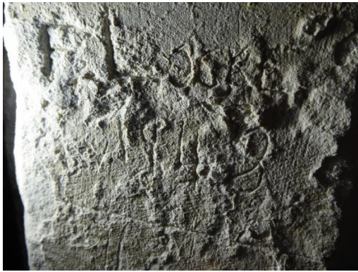
Fig 19. Clock chamber door jamb. F Locke 1948
