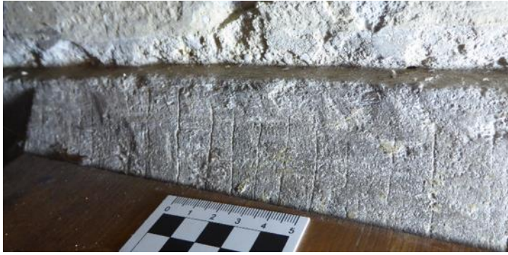
Fig 48. North of chancel arch. Vertical lines scratched into stonework next to pulpit steps
