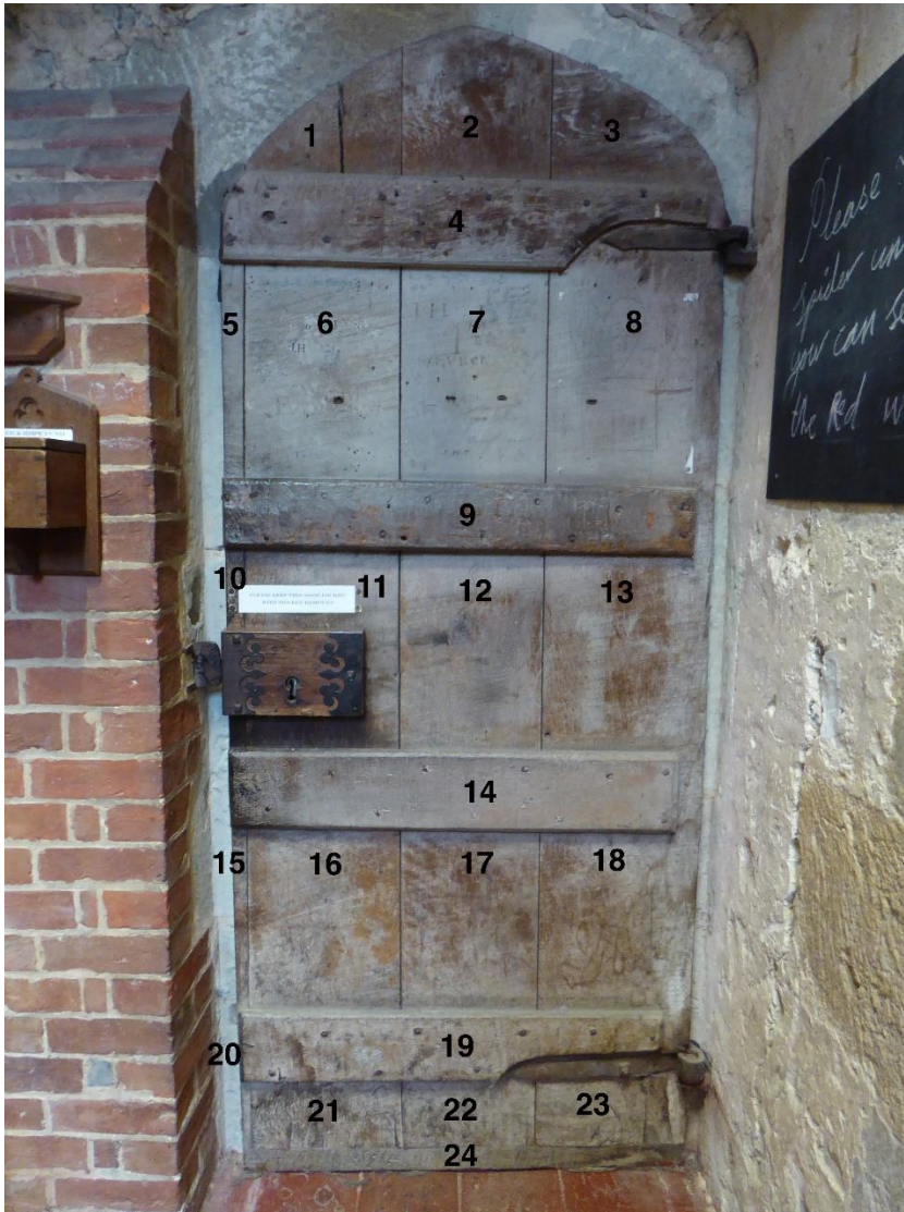
Fig 37. Ringing chamber. Main door, with numbered panels
