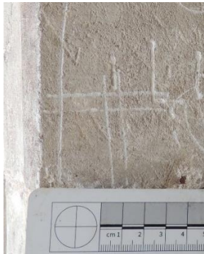
Fig 6. South inner doorway. Modern cross
