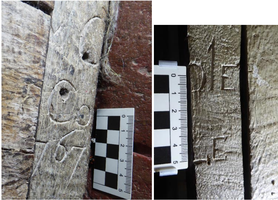
Figs 38 & 39. Ringing chamber. Main door. Reused timbers, door panels 24 and 5, with partial date 1767 and lettering
