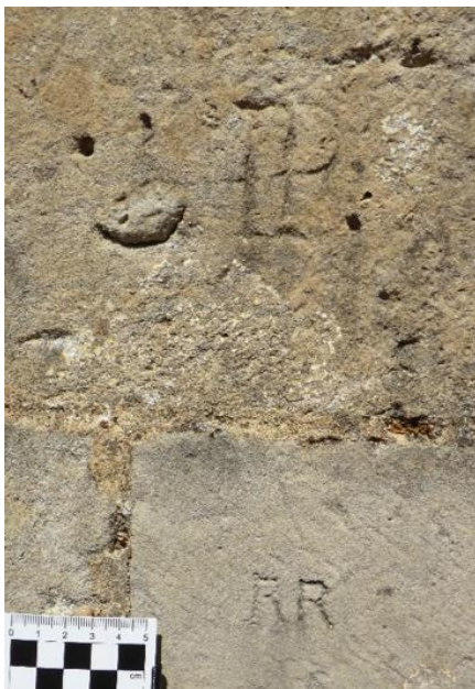
Fig 78. South wall of nave. Pairs of initials
