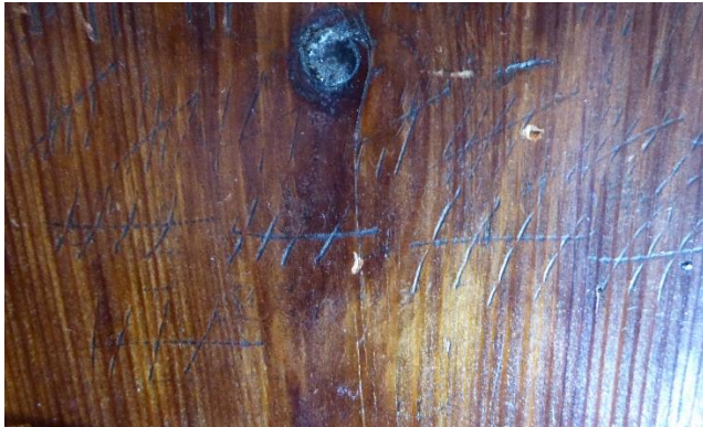
Fig 36. Ringing chamber panelling. Tally marks
